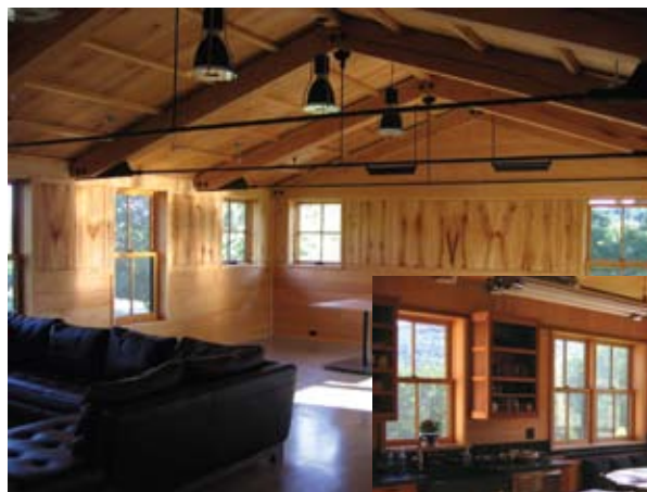
Above Left: Scott Burt of Topcoat Finishes. Below: Topcoat did all the painting in this model of sustainable building practices. The substrates were predominantly maple and cherry woods, plaster and a small component of drywall. Bioshield oil was applied to all the wood surfaces, with Benjamin Moore Aura on the paint grade elements.
