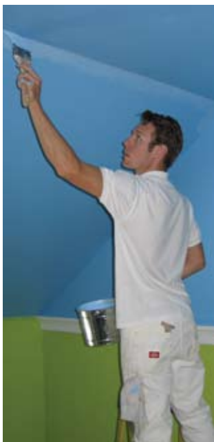
By learning to cut in this painter saves on tape.
